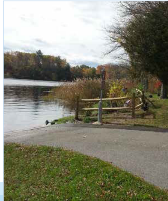
New streambank restoration and planting has transformed this once heavily eroded access point.
