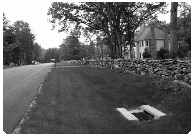
Storm low impact design in a local subdivision. Photo courtesy of CRCCD.
