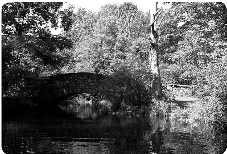
East Branch Eightmile Mumford Farm Crossing. Photo courtesy of L. Todd.
