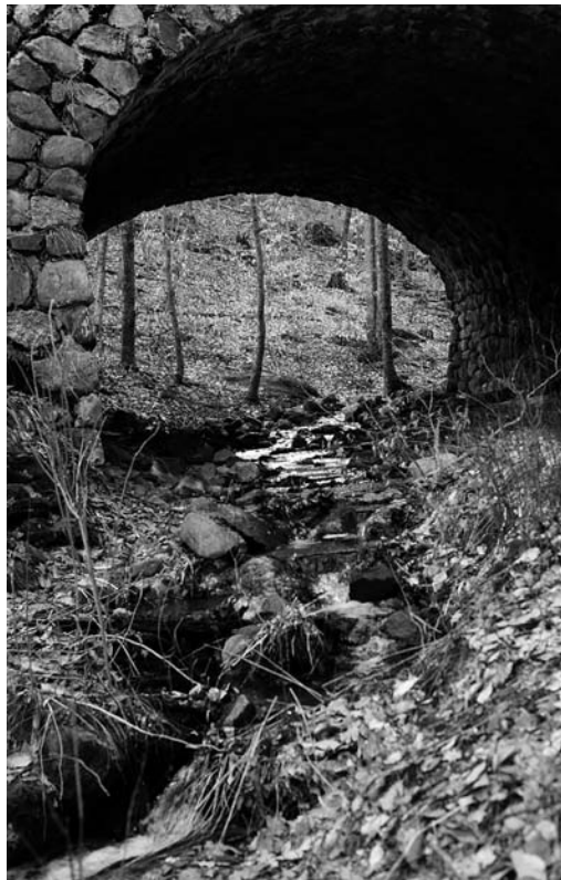
Stream Crossing in East Haddam
