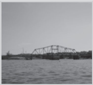
Photo: Historic Berkley-Dighton Bridge.
