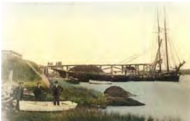
Historic Post Card of Pottersville Wharf on the Taunton River in Somerset
