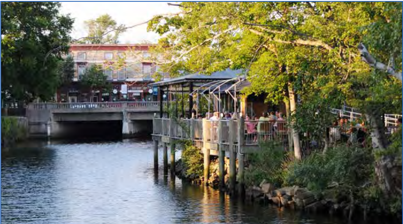
Rt. 1 bridge over the Pawcatuck River, Westerly, RI/Pawcatuck, CT (Photo credit: Dan Hyland)
