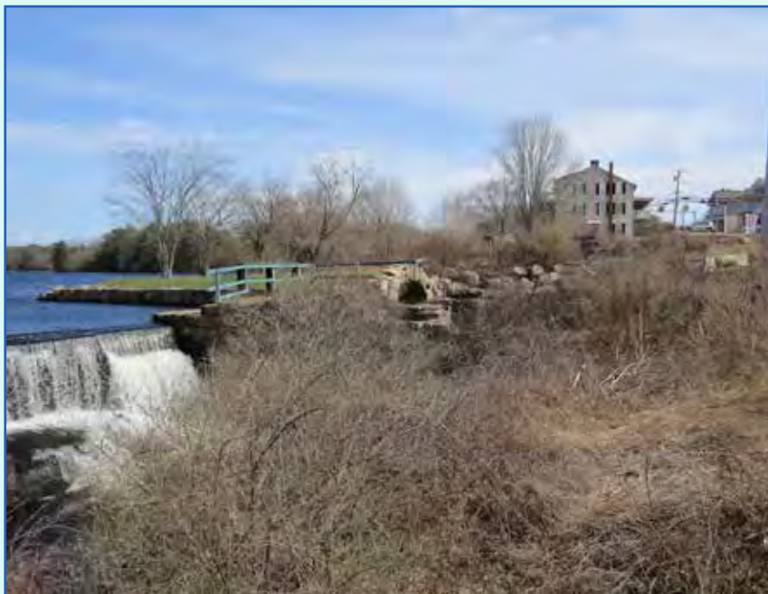
Wyoming Dam in Richmond, RI (Photo credit: Elise Torello)
