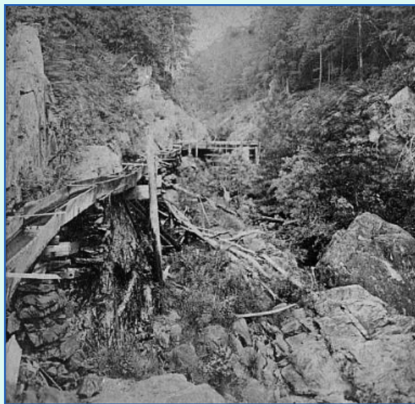
1875 photo by M. Herbert Kenyon of a wooden sluiceway held up on rock cairns across Green Fall River ravine, Voluntown, CT.
