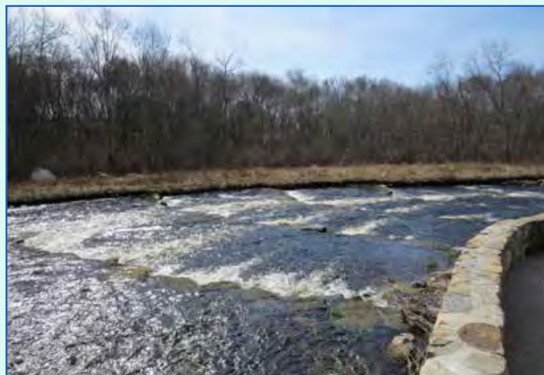
Nature-like fish passage in the Pawcatuck River at Kenyon Industries, Charlestown/Richmond, RI (Photo credit: Elise Torello)
