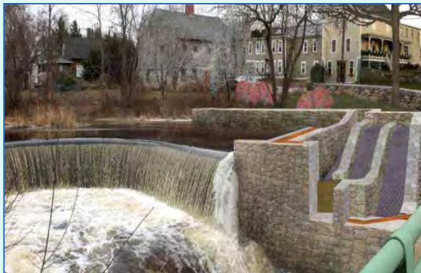
Fish and eel passage at Horseshoe Falls on the Pawcatuck River, Charlestown, RI (Photo credit: Denise Poyer)
