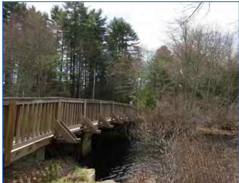
Dugway Rd. bridge on the Queen River, South Kingstown, RI (Photo credit: Elise Torello)
