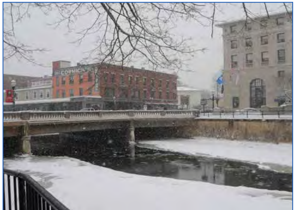
Rt. 1 bridge over the Pawcatuck River, Westerly, RI/Pawcatuck, CT (Photo credit: Dan Hyland)
