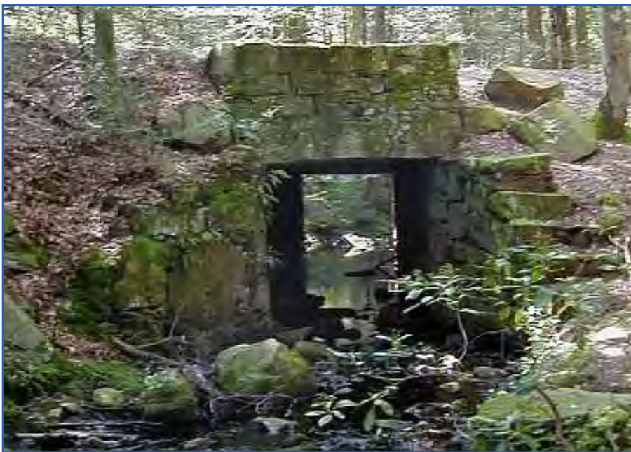
Green Fall bridge, North Stonington, CT (Photo credit: David R. Brierley
