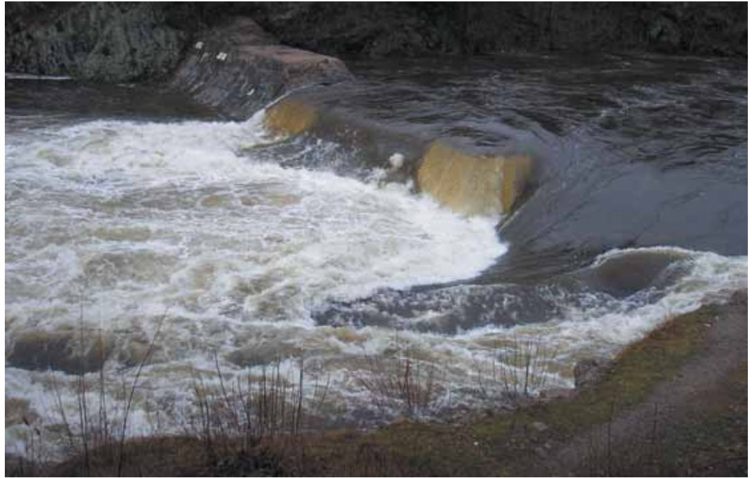
Spoonville Dam Photo: Joyce Kennedy
