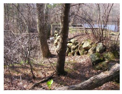
Most traces of the mill buildings are long gone. Water channels and stone foundations persist — artifacts that nature has not yet reclaimed completely. Pictured here is the original stone and earth dam at the site of Dawley's grist mill, later owned by the Hall brothers. A modern concrete structure now regulates water flow.
